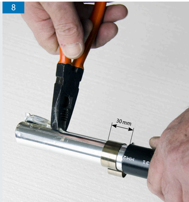
Removing the unnecessary armouring tape to ensure the insulation distance between cable lug an armouring / screen.
