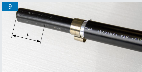
Strip the insulation in the length "L" according to the cut back dimensions mentioned in the instruction of the cable lug.
